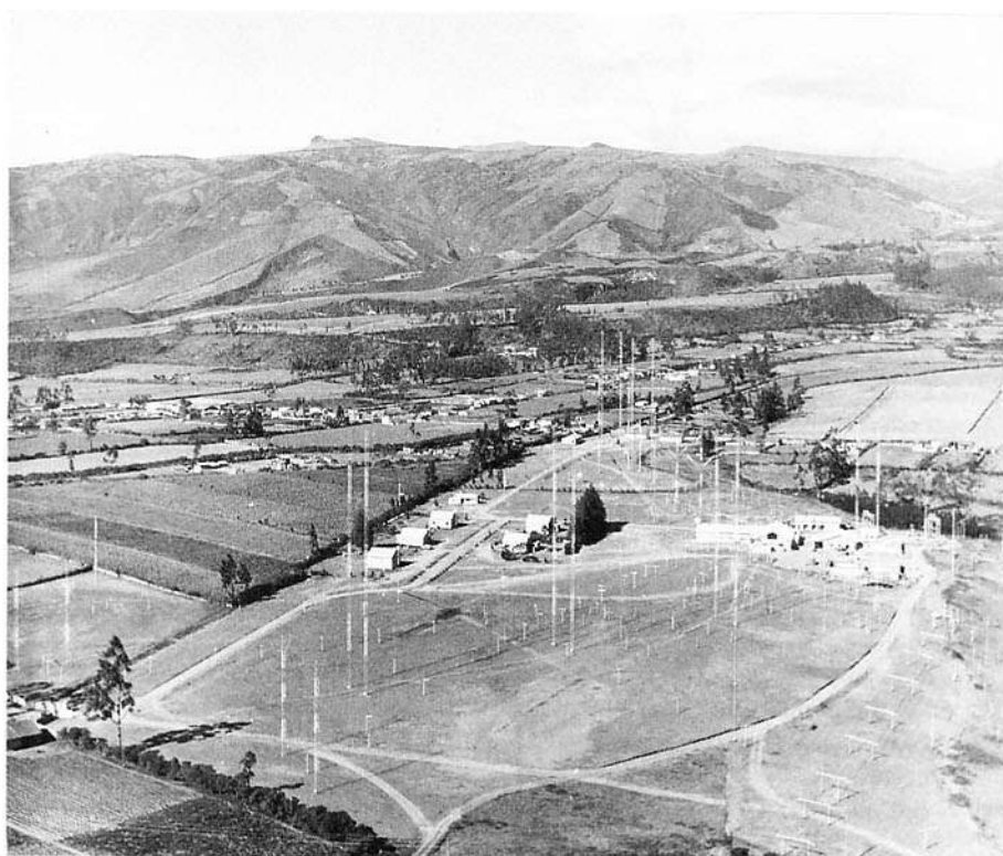
Fig 1—Radio heaven or radio hell? The antenna system of HCJB, near Quito, Ecuador, was located literally in the author's backyard! His house is at the center of the photo, the top building in the row of four.
